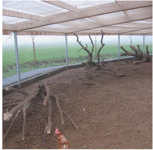
Figure 6- example of a veranda with a timber roof frame and plastic sheets as roof cover.
