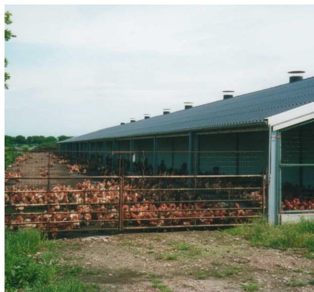
Figure 2 - lean to/awning style veranda with sloping roof and metal sheets on the roof. This example has side walls made of wire
