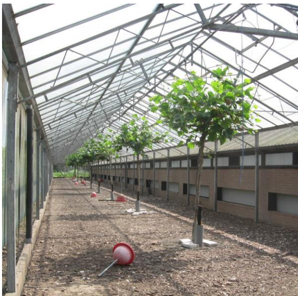
Figure 7- example of a veranda with a steel roof frame and plastic sheets as roof cover.
