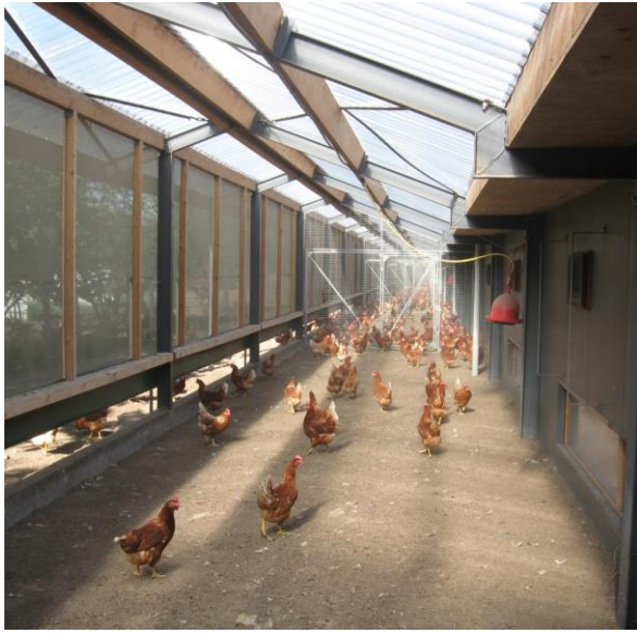
Figure 5- example of a veranda with a roof frame built from steel and wood and plastic sheets as roof cover.
